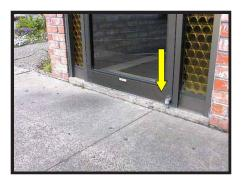
Step 2. Determine the type of Landing and approach your application requires. There are three basic types of Landing configurations: one-sided, two-sided and three-sided approaches. Three-sided Landings are the most popular variety as they allow for three sides of approach into the facility. There are instances where structural impediments exist such as walls, planters or curbing which makes one-sided or two-sided Landings the better option.
